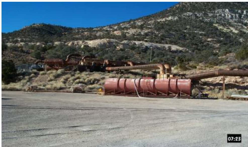
Figure 5-7. U12g Tunnel 16,000-gallon water tank.
