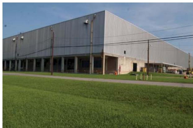
Southeast Corner of the K-29 Building
