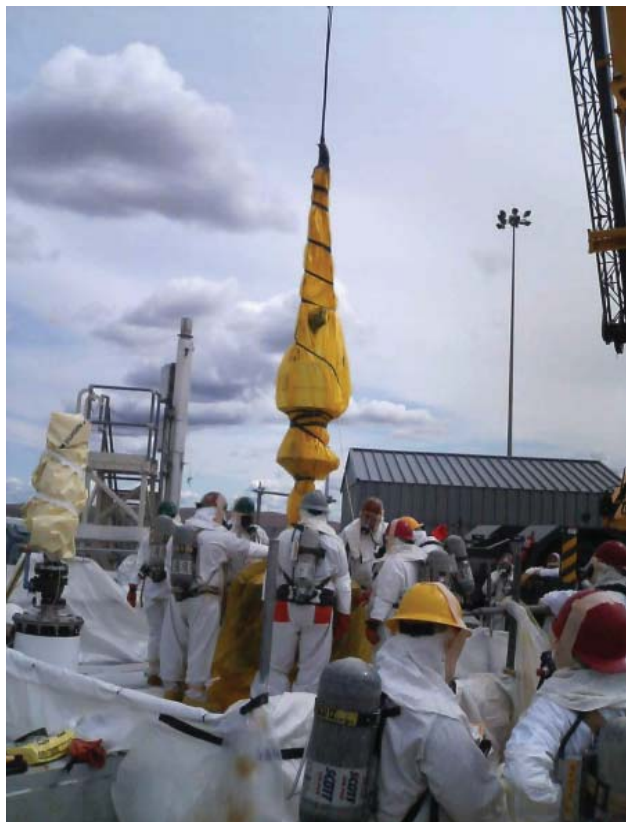
Removing a Failed Slucicer at Tank C-103
