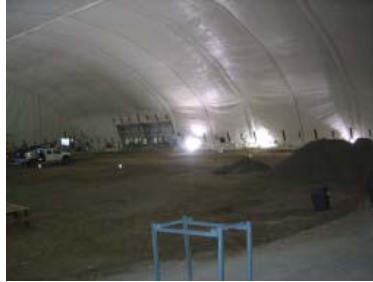
Accelerated Retrieval Project 2 Construction
