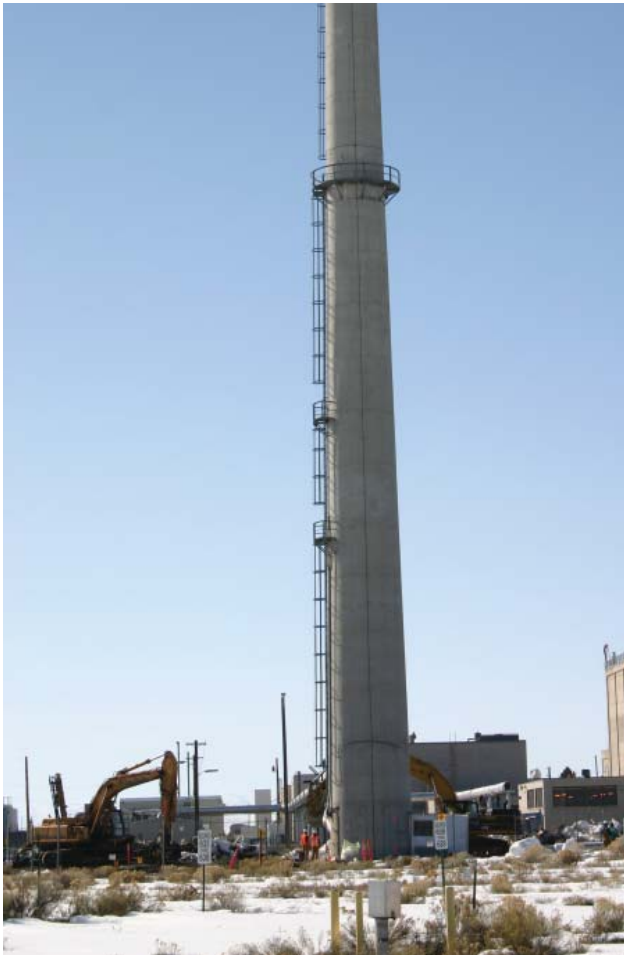
Preparations to Demolish the Engineering Test Reactor Stack
