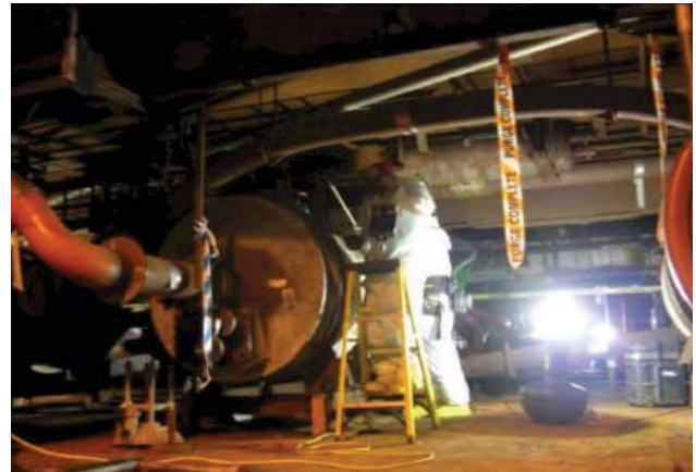
Vent/Purge/Drain Activities in K-25 Building
