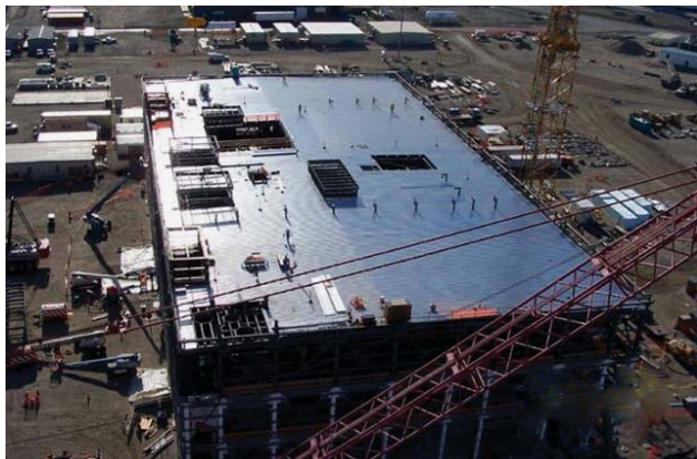
Prepping Roof on Low Activity Waste Facility
