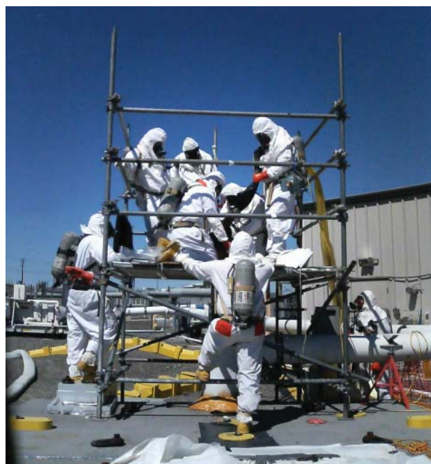
Replacing an In-Tank Video Camera in Tank C-103 To Support Waste Retrieval Activities
