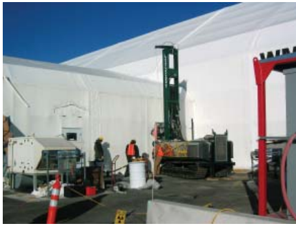
Accelerated Retrieval Project Foundation Stabilization
