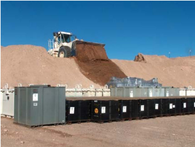
Glovebox Burial. The Low-Level/Mixed Low-Level Waste (LLW/MLLW) Project Facilities Located in Area 5 of NTS Provide Disposal Services for On-Site and Off-Site DOE Generators
