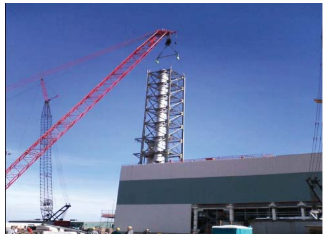
Setting of Low Activity Waste Facility Stack
