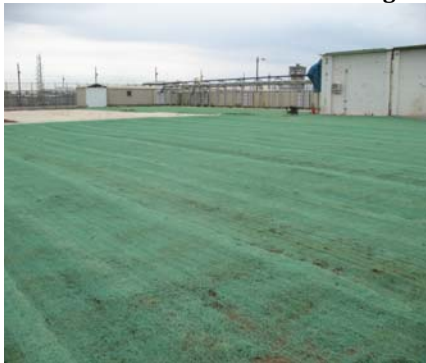
After Demolition of Building 12-9
