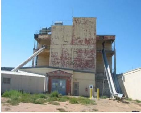
Before Demolition of Building 12-9
