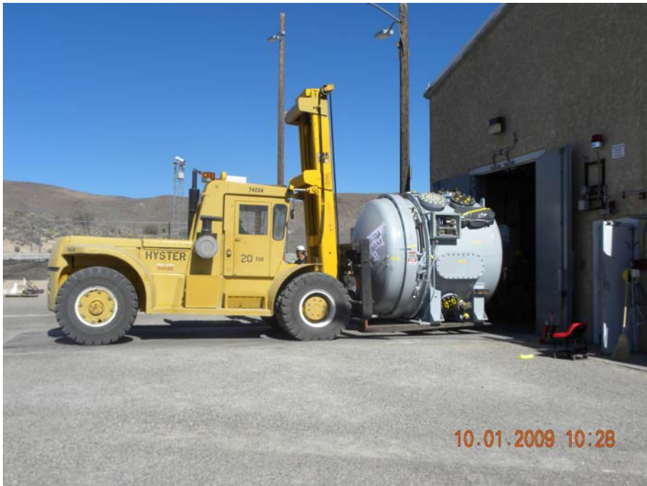
Replacement of the JASPER Facility secondary confinement chamber
