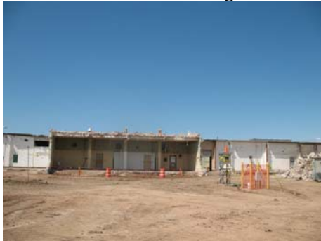
Mid-Point of Demolition of Building 12-9
