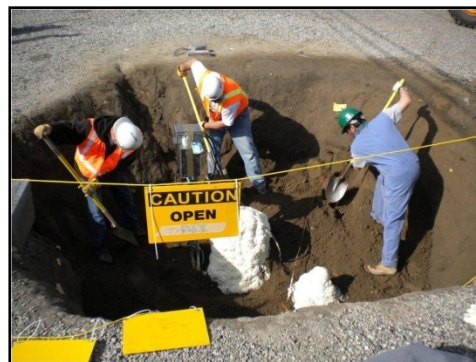
Tank Farms workers remove Clean Out Boxes (COB) at the AW farm.
