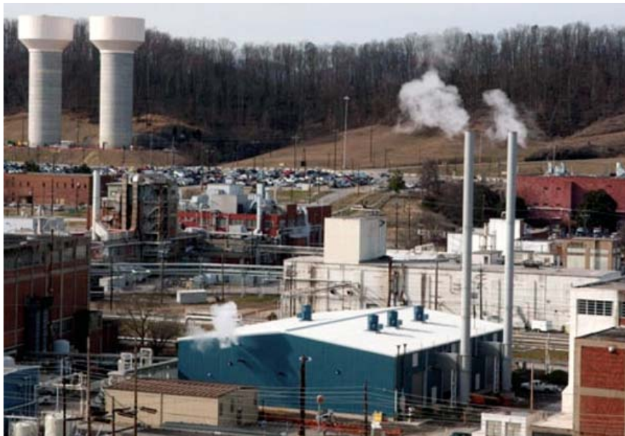
New Y-12 steam plant with Chestnut Ridge water tanks in the background
