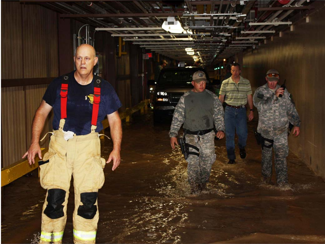
Rainwater Flooding in Ramps at Pantex Plant
