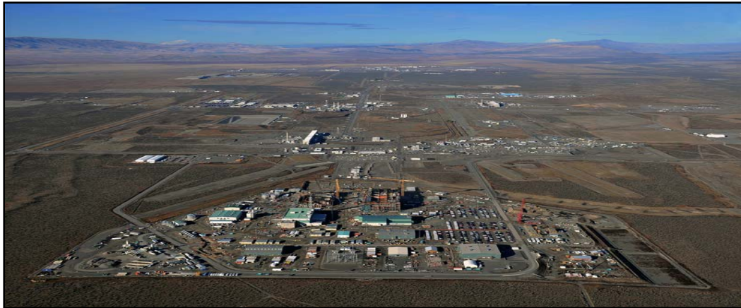
Hanford Waste Treatment and Immobilization Plant and Tank Farms, October 2010
