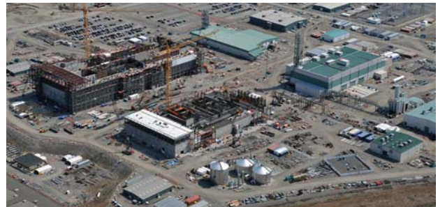
Hanford Site's Waste Treatment and Immobilization Plant
