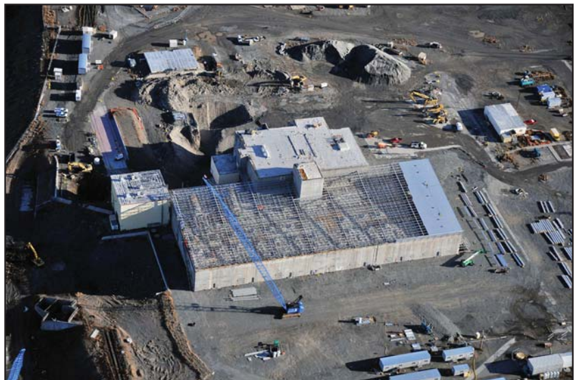
DOE Nuclear Facility Construction Project
