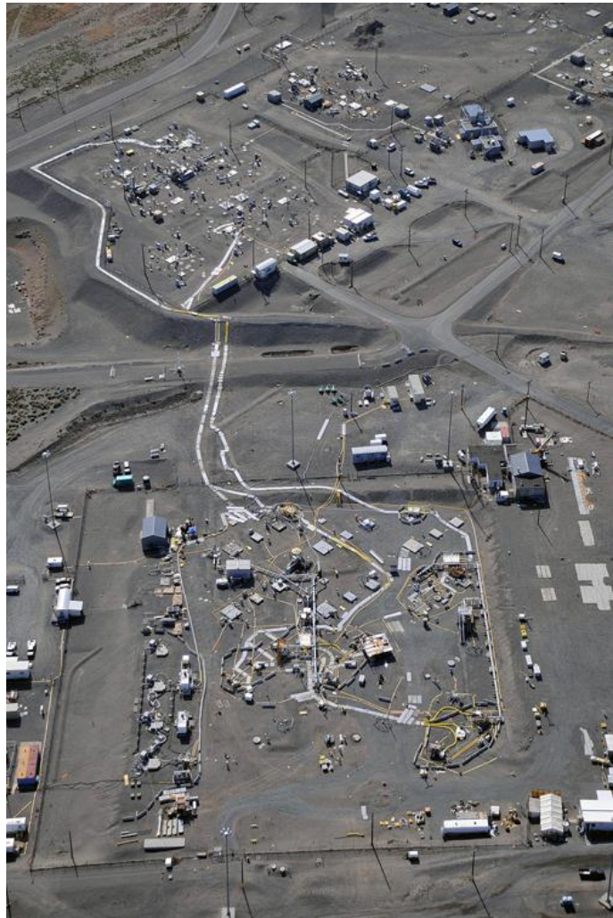
Hanford Tank Farms Aerial View
