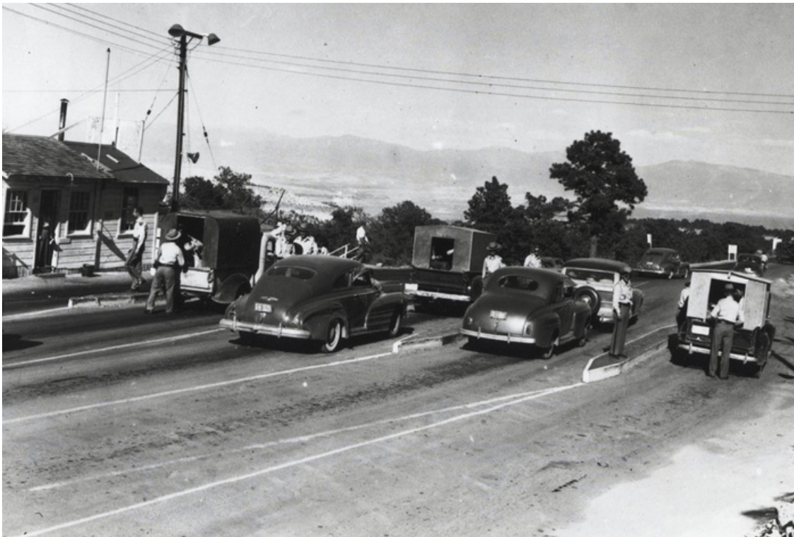
Los Alamos Main Gate, Manhattan Project
