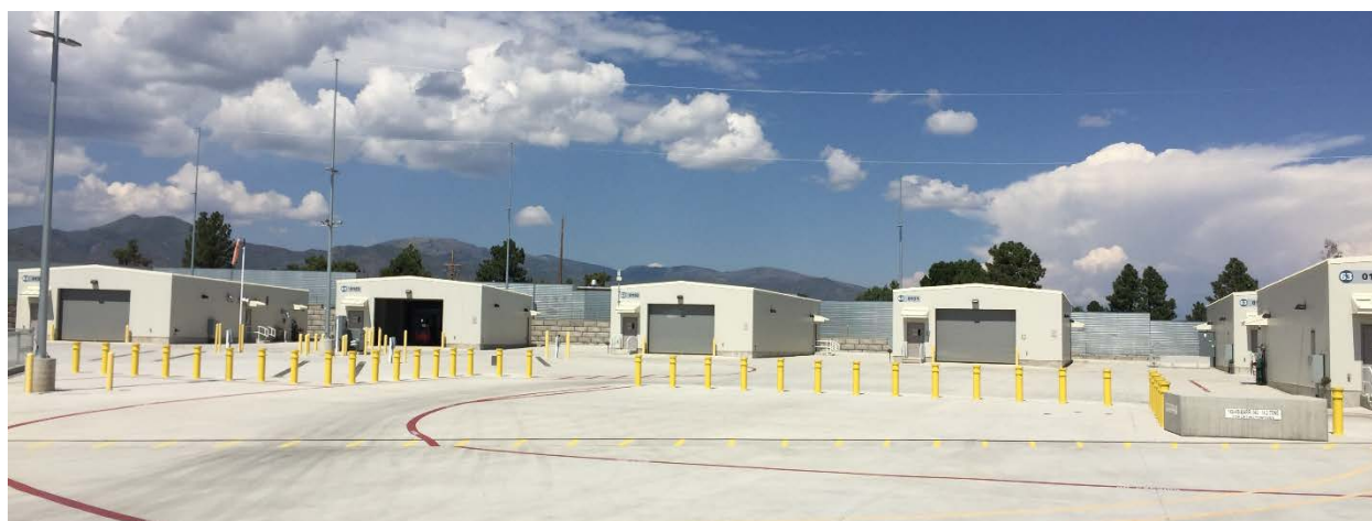
Figure 1 – Completed Transuranic Waste Facility
