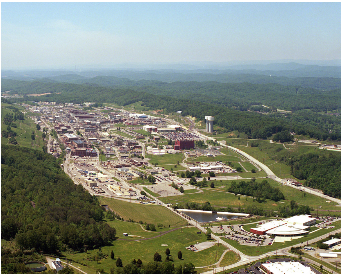
Y-12 National Security Complex
