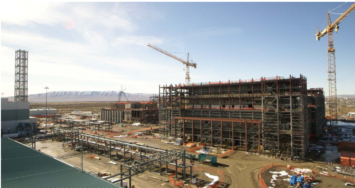
Waste Treatment and Immobilization Plant, Hanford Site
