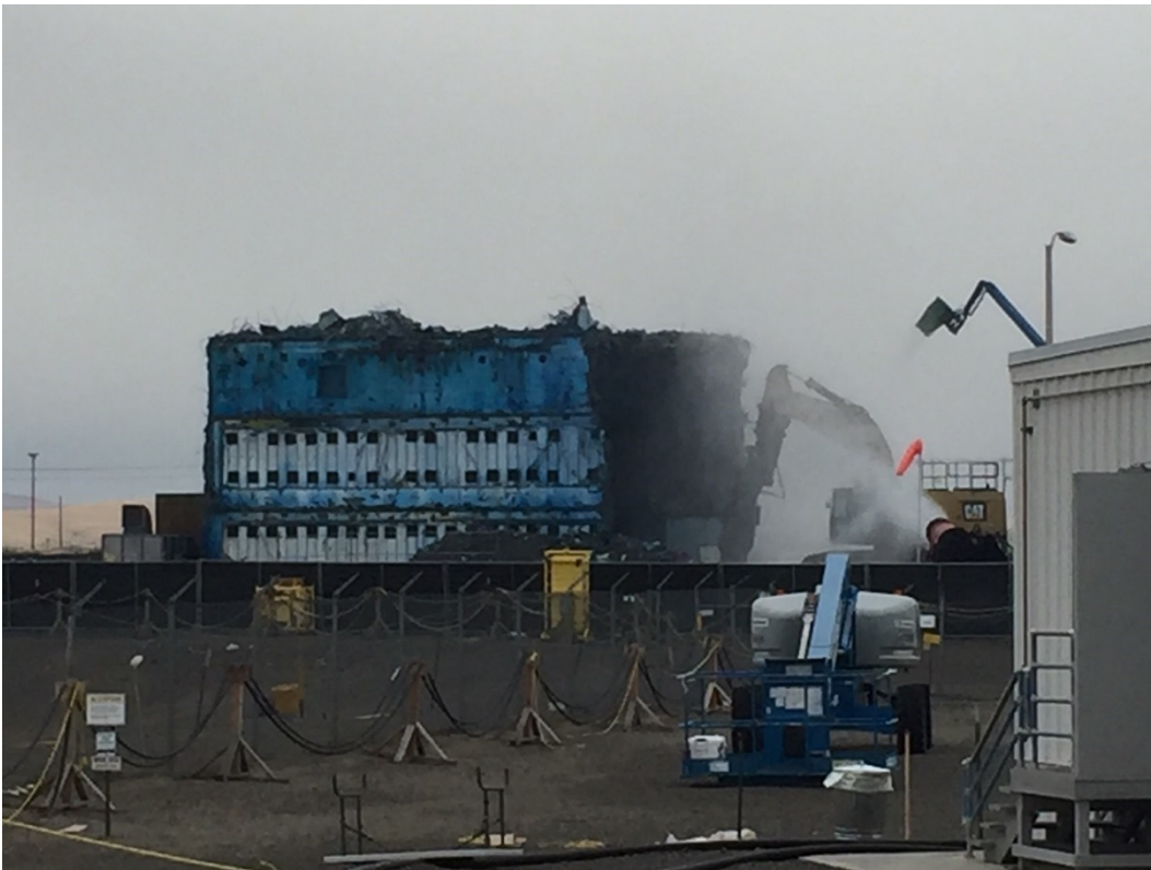
Demolition of the Hanford Plutonium Finishing Plant
