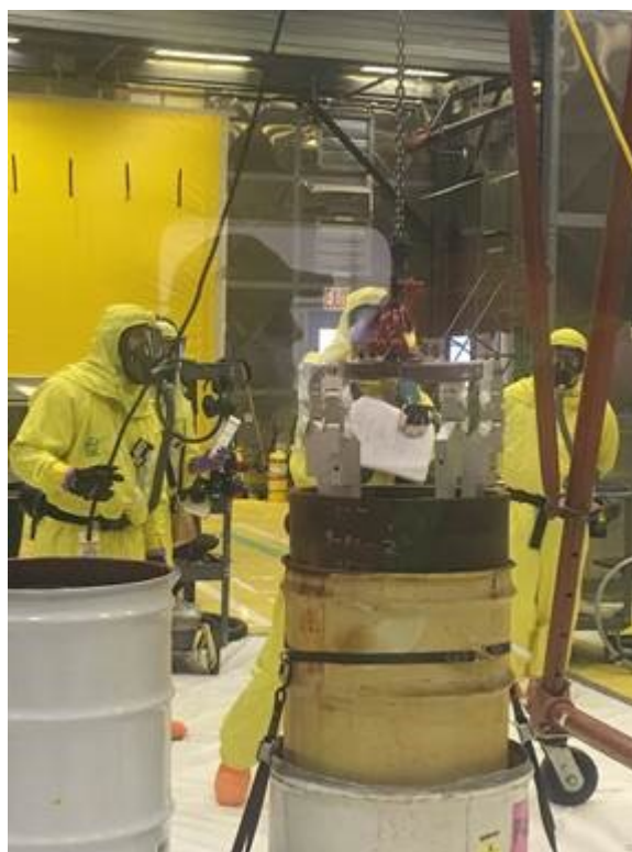
Unremediated Nitrate Salt Waste Processing at LANL
