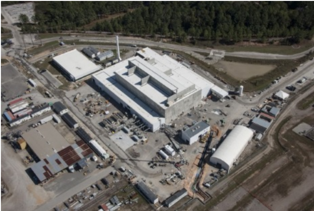
Salt Waste Processing Facility, Savannah River Site
