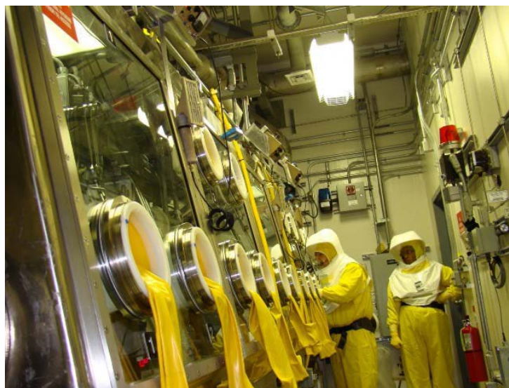
K-Area Complex Glovebox Operations
