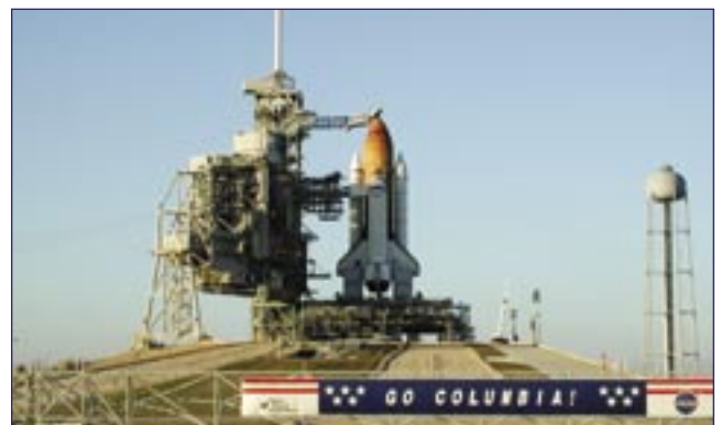
Figure 2.1-1. Columbia, at the launch pad on January 15, 2003.
