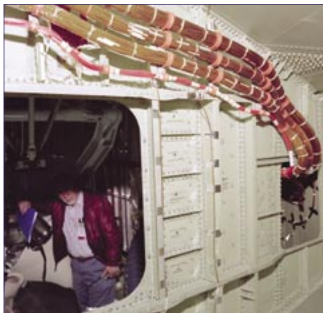
Figure 4.2-3. Typical wiring bundle inside Orbiter wing.
